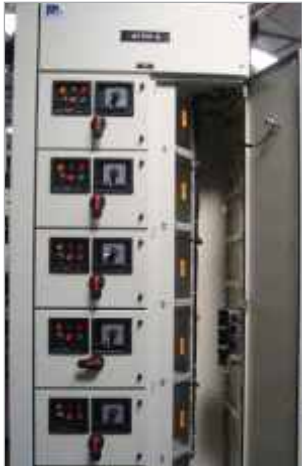
Foam- 4, Type - 7 construction
